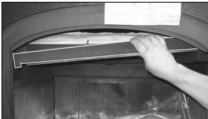
Figure 4.5 Removing Baffle Protection Channel
