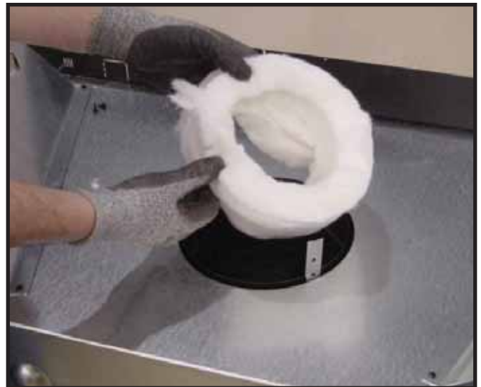
Figure 9.5 Remove the insulation from the outer vent pipe. For rear venting there is no insulation in the outer vent pipe.
