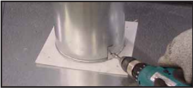
Figure 9.6 To attach the first section of vent pipe, make sure to use the fiberglass gasket in the manual bag to seal between the first vent component and the outer fireplace wrap. Caulk with a minimum of 300°F continuous exposure rating may be used to hold the part in place.
