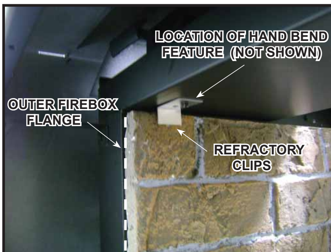
Figure 11.15 Refractory Clip Installation
