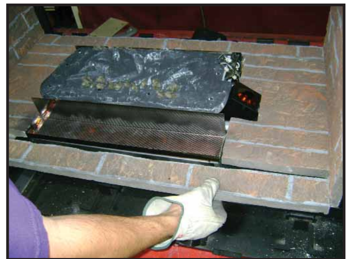
Figure 11.18 Positioning Outer Bottom Refractory.
