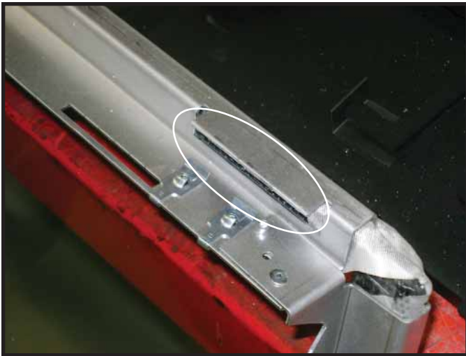
Figure 11.1 Glass Top Tab Detail.
