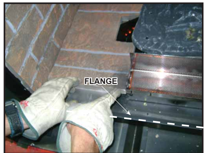
Figure 11.17 Positioning Left and Right Middle Base Refractory
