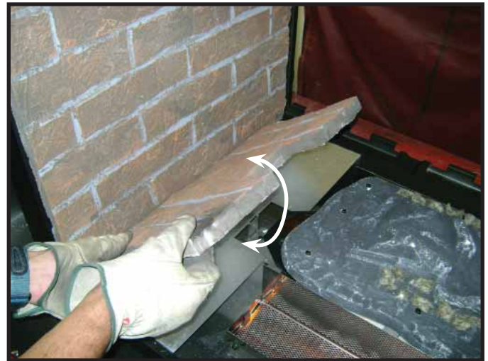
Figure 11.16 Positioning Inner Bottom Refractory
