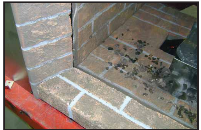
Figure 11.27 Outer Hearth Installation
