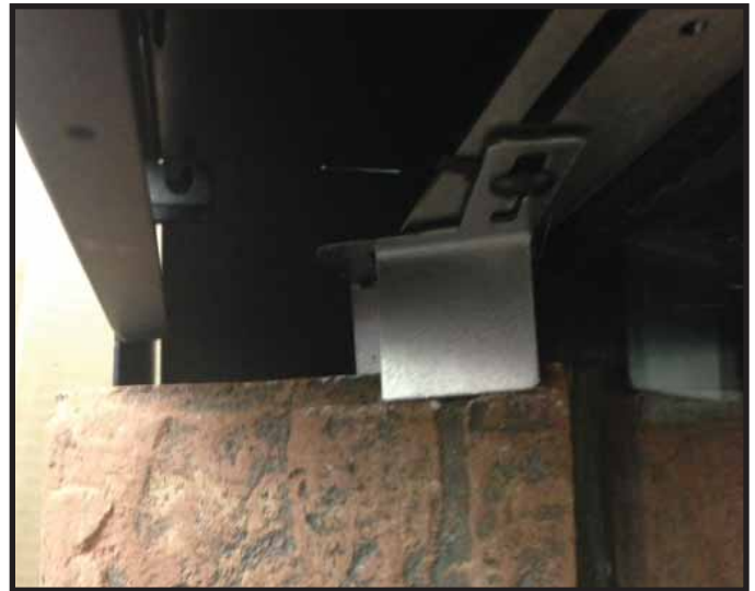
Figure 11.26 Side Refractory Brackets
