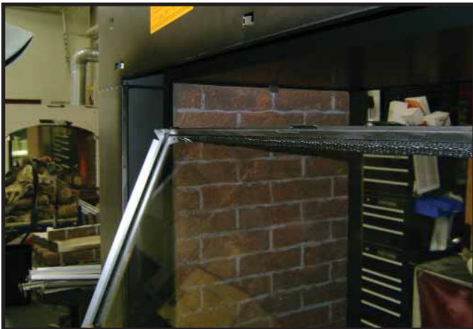
Figure 11.2 Initial Positioning of Frame into Opening.
