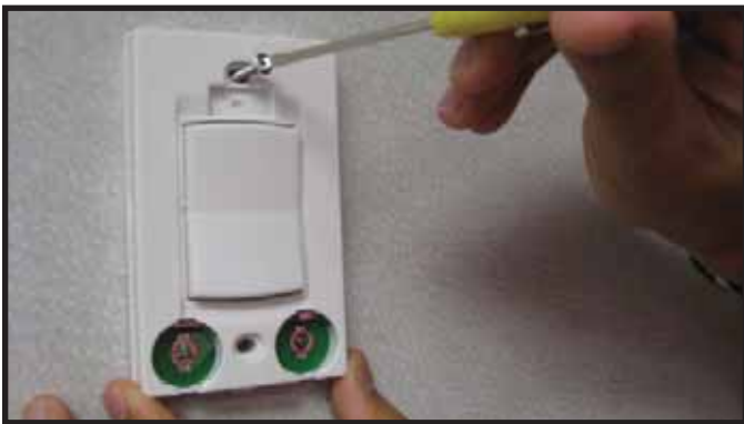
Figure 2. Mounting Wireless Wall Switch
