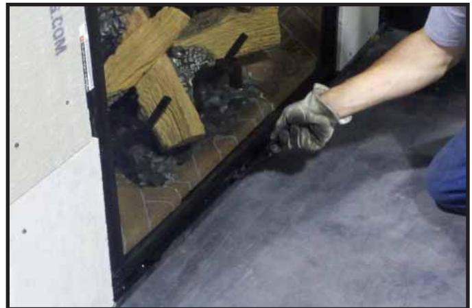
Figure 11.8. Securing Bottom Glass Clips
