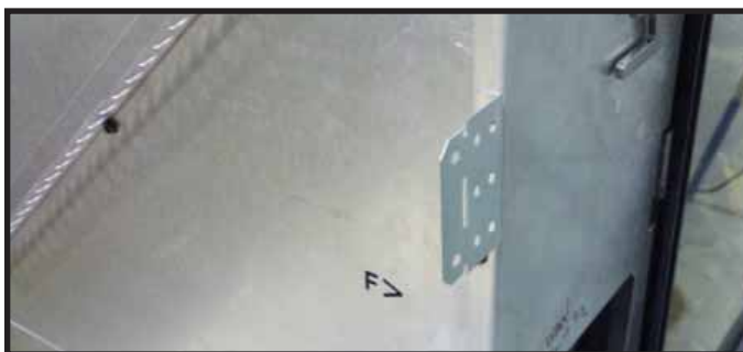
Figure 6.5 Nailing Tab Bent Out for Installation
