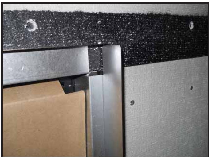
Figure 10.5 Finishing Template Bends
