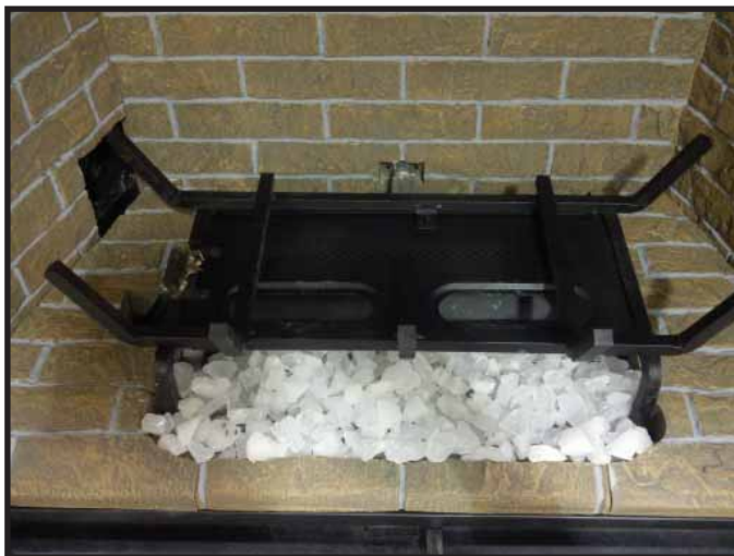
Figure 11.20. Ember Glass Area Covered with Teco-Sil
