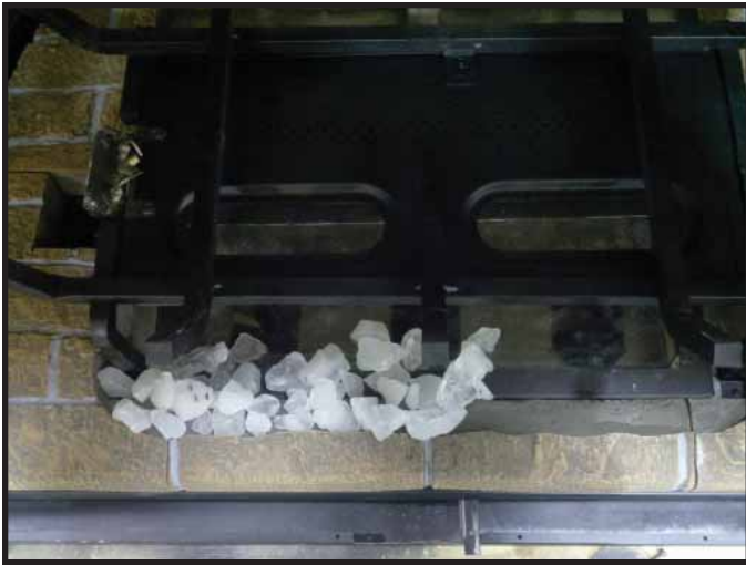
Figure 11.19. Install Teco-Sil
