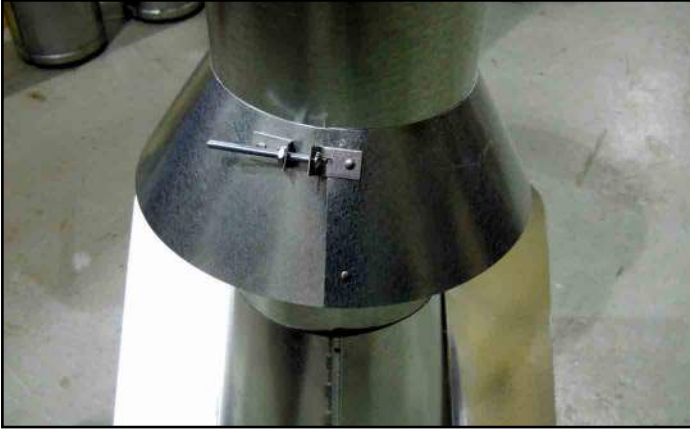
Figure 7.14 Insert Bolt into Brackets
