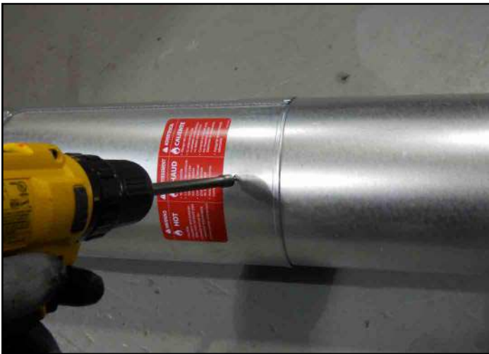
Figure 7.4 Screws into Slip Section
