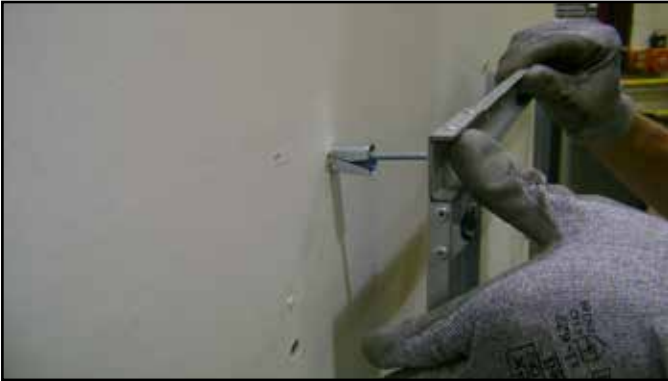
Figure 4.6 Installing Anchors in Hollow Wall
