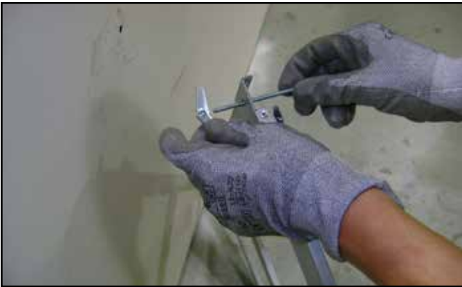
Figure 4.5 Toggle Bolt Installation through Mounting Bracket
