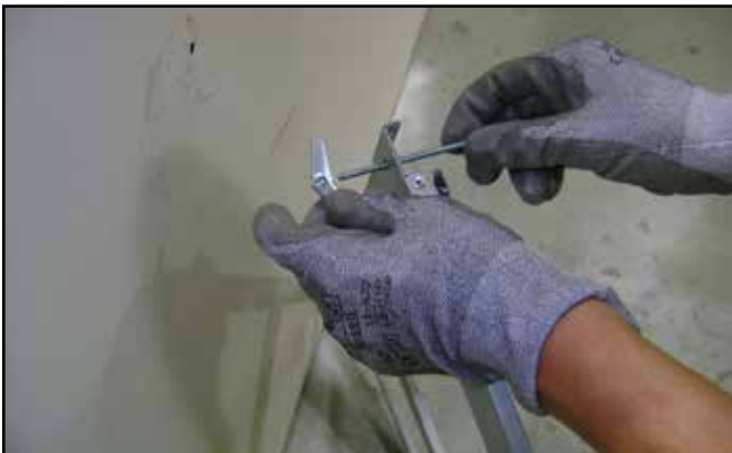
Figure 4.5 Toggle Bolt Installation through Mounting Bracket
