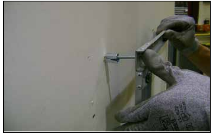
Figure 4.6 Installing Anchors in Hollow Wall
