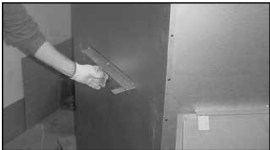
Figure 3.6 Bend Refractory Brackets Back Down
