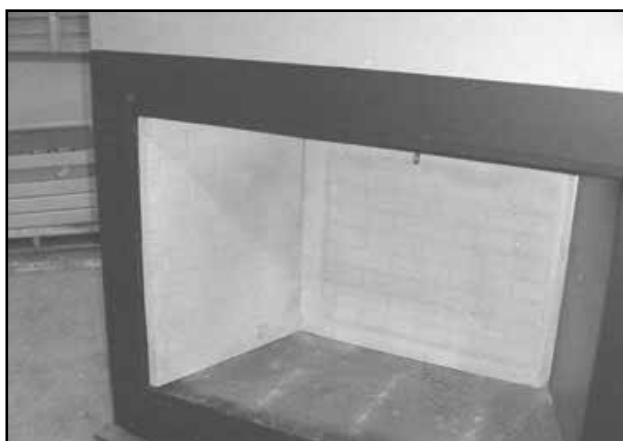
Figure 8.6 Side Refractory Installed
