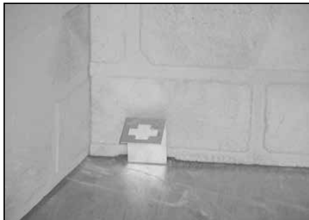
Figure 8.8 Grate Retaining Bracket in Place
