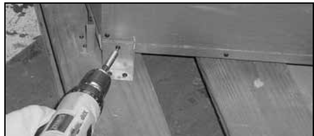
Figure 3.10 Removing Shipping Brackets
