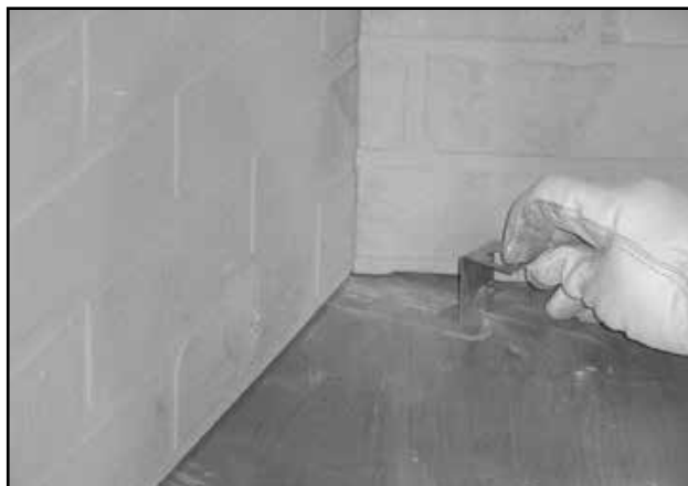
Figure 8.7 Slide Grate Retaining Bracket into Notch
