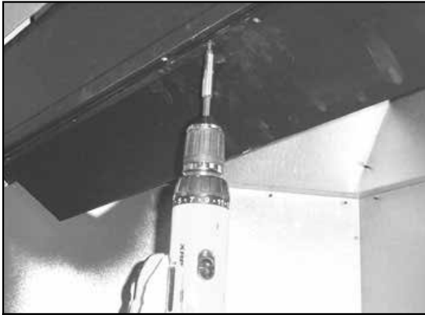
Figure 8.1 Remove Smoke Shield
