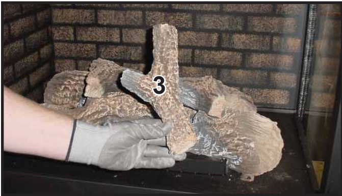
Figure 13. Placement of Log #3
