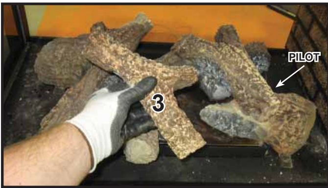
Figure 7. Placement of Log #3
