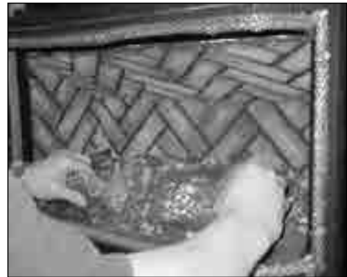
Figure 6.2 - Lift burner up and out of the firebox opening.
