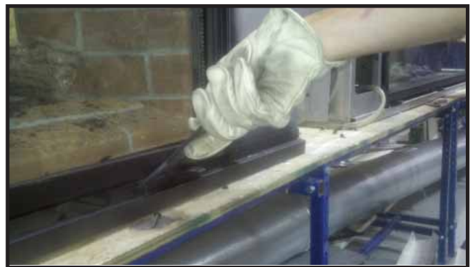
Figure 11.3 Inserting Glass Clip Tool
