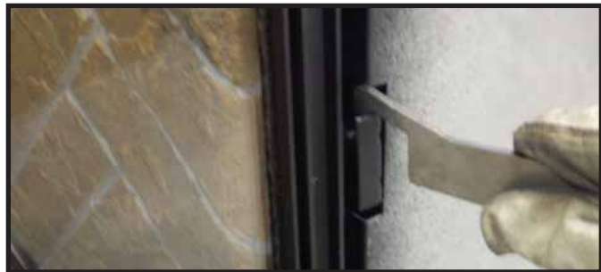
Figure 11.7. Fasten Side Glass Clips
