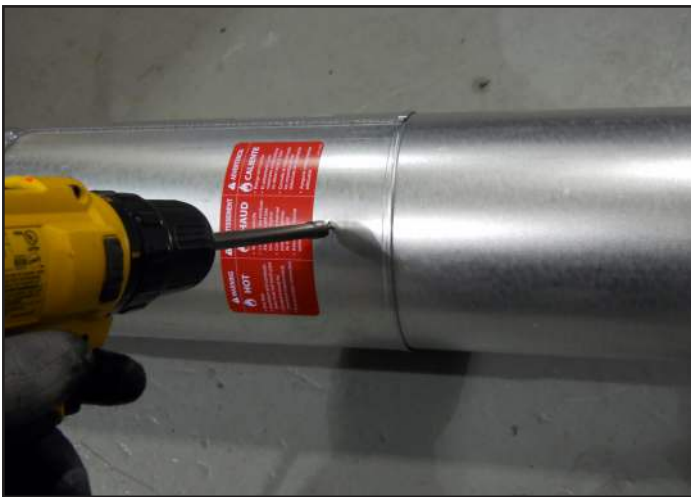
Figure 7.4 Vis de la section coulissante
