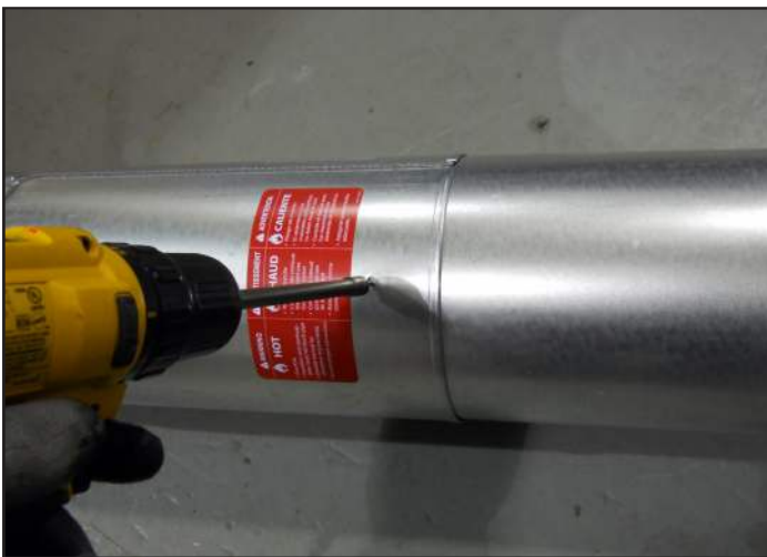
Figure 7.4 Vis de la section coulissante
