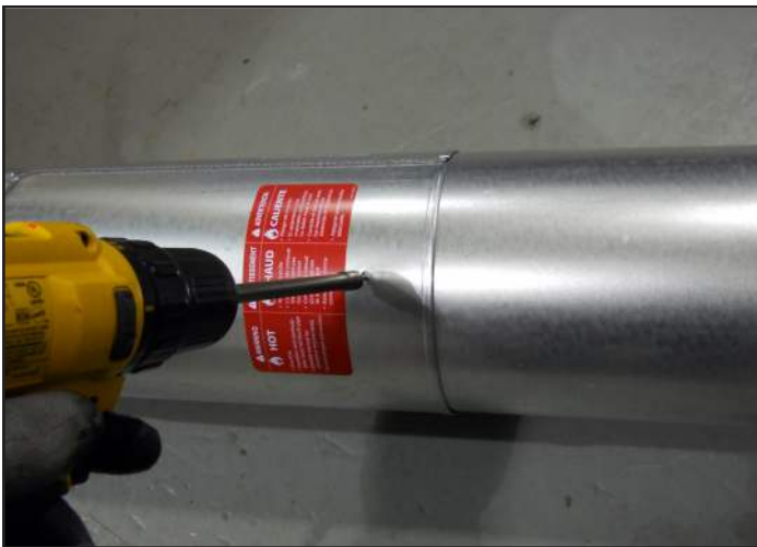
Figure 7.4 Vis de la section coulissante
