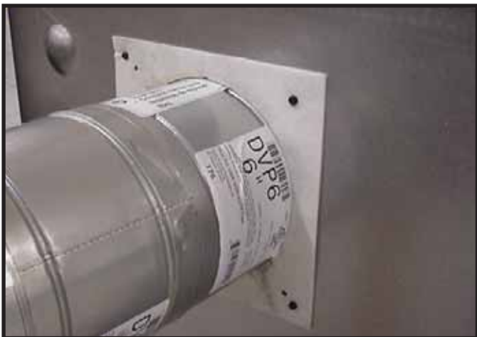
Figure 9.16 Attach the first vent section (it will snap into place). Slide the insulation gasket onto the vent section, up against the appliance and over the tabs. Use two self-tapping screws to secure gasket to outer wrap.
