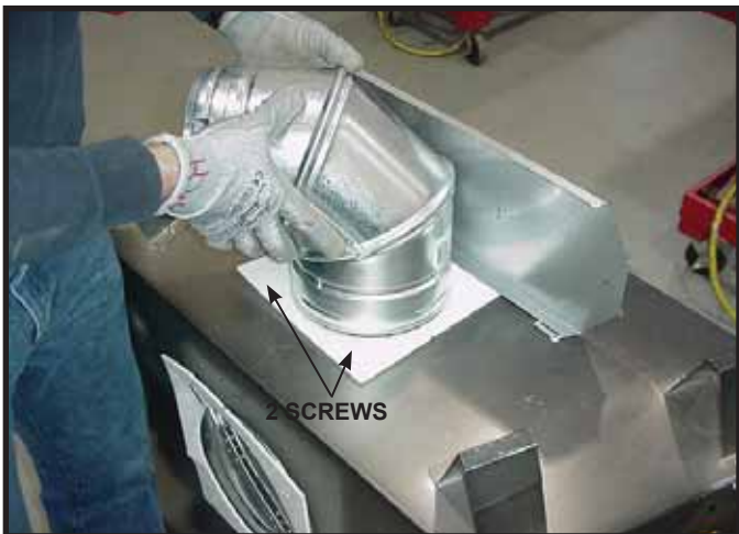
Figure 9.9 To attach the first section of vent pipe, make sure to use the fiberglass gasket to seal between the first vent component and the outer fireplace wrap. Use 2 self tapping screws to secure the gasket to the outer wrap.
