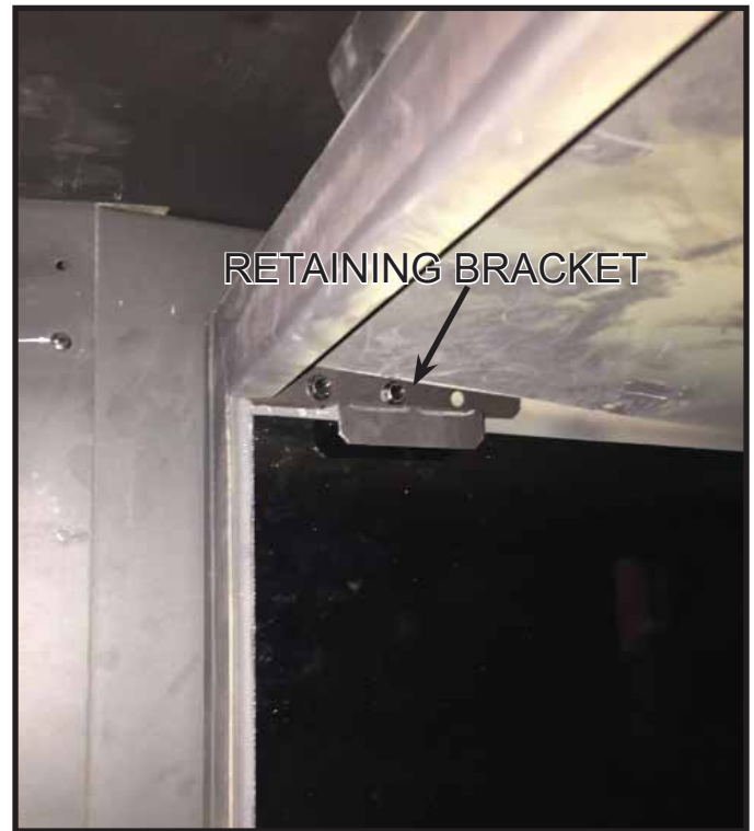
Figure 11.5. Retaining Bracket Installation - Single-sided Models
