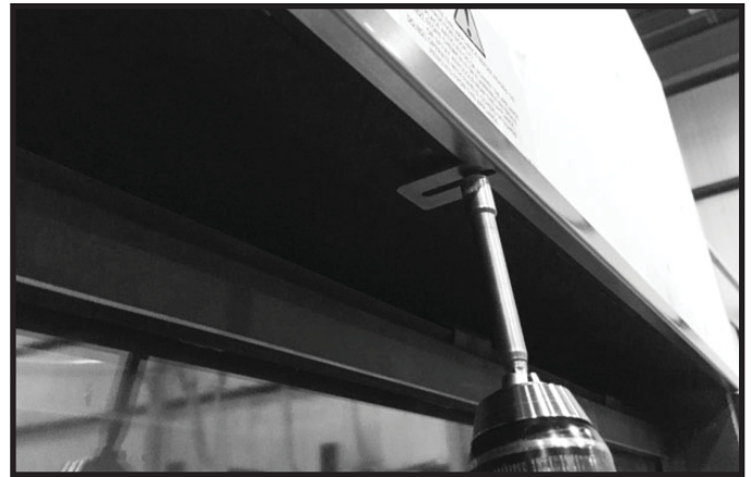
Figure 10.5. Install Trim Ring
