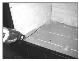
**Figure 10.3**. Using a saws-all, cut out the floor.
