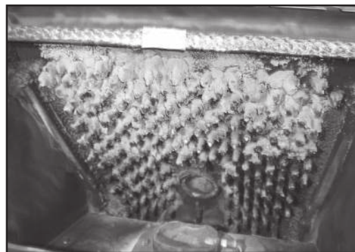
Figure 23.2 - Example of a dirty heat exchanger
