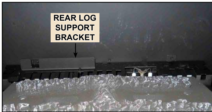
Figure 10.4 Install Rear Refractory
