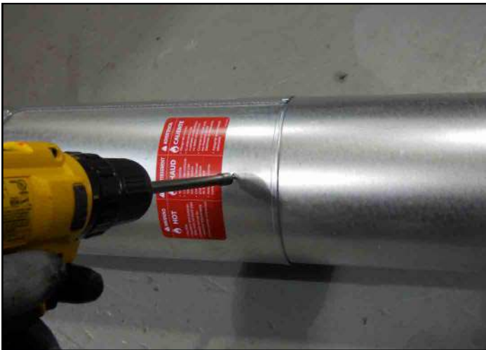
Figure 7.4 Screws into Slip Section
