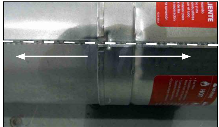
Figure 7.8 Align and Disassemble Vent Sections
