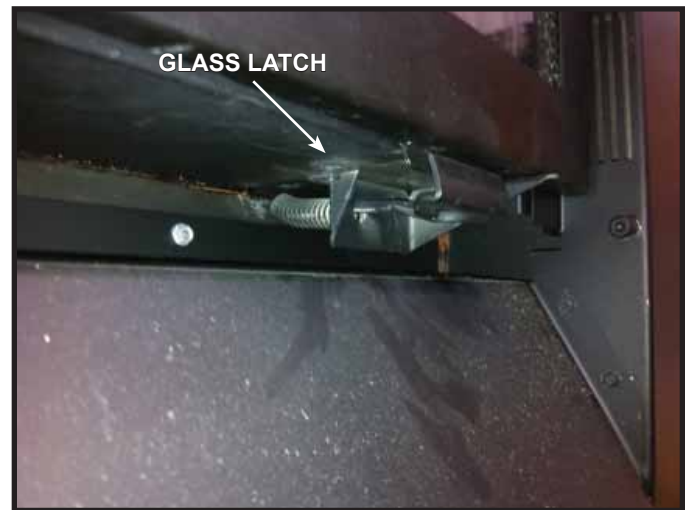
4.4 Glass Latch Detail - Exterior Side
