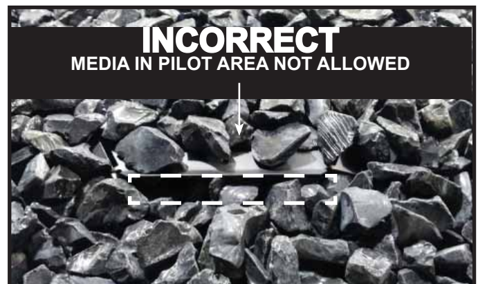
Figure 9.7 INCORRECT Media Placement
