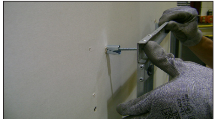
Figure 4.10 Installing Anchors in Hollow Wall
