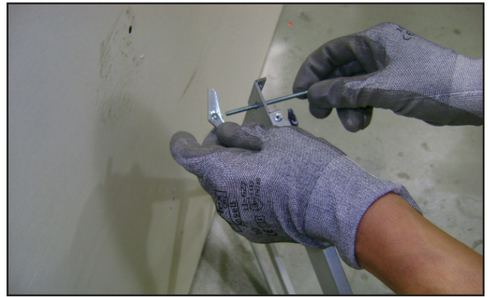
Figure 4.9 Toggle Bolt Installation through Mounting Bracket
