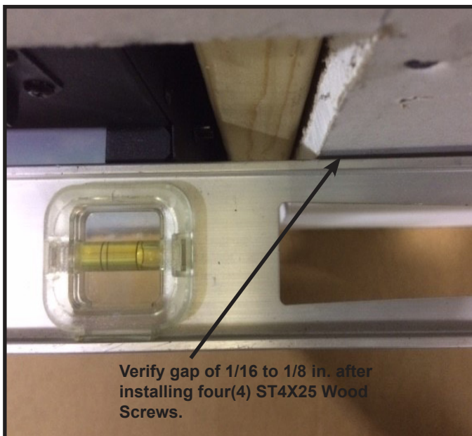
Figure 4.5 Adjust Bracket Location
