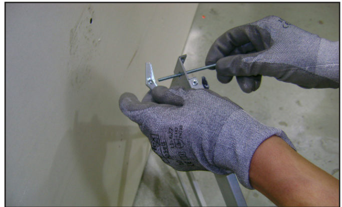
Figure 28. Toggle Bolt Installation through Mounting Bracket
