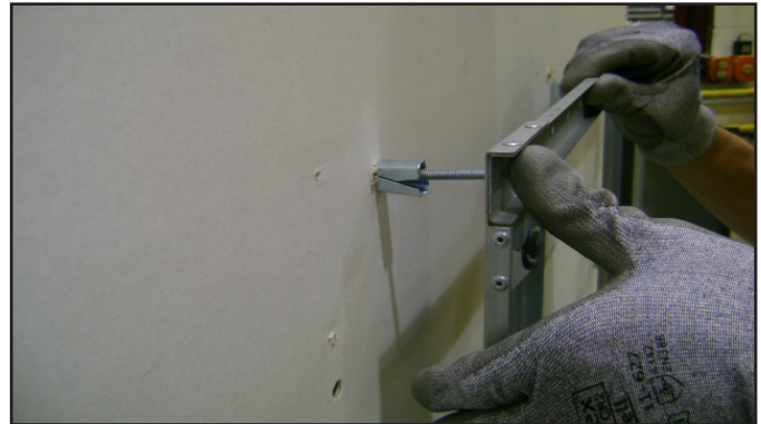
Figure 29. Installing Anchors in Hollow Wall
