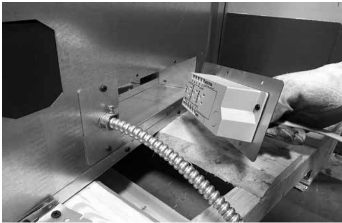
Figure 8.5 Junction Box Assembly
