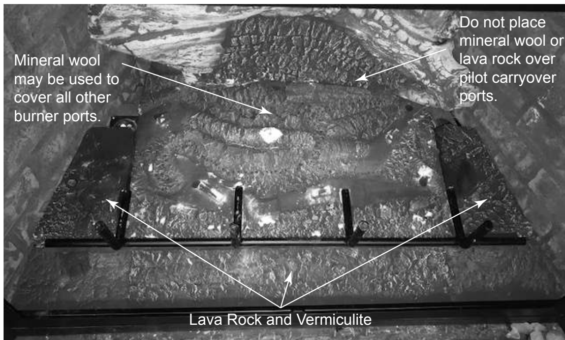
Figure 11.17 Placement of Mineral Wool, Lava Rock and Vermiculite
