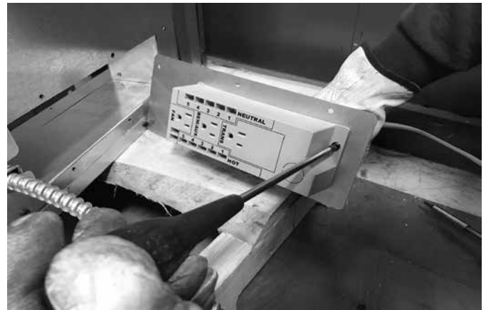
Figure 8.6 Junction Box Removal
