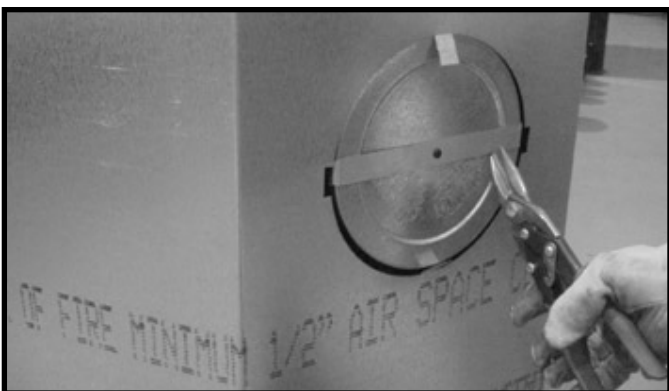
Figure 6.8 (Generic Fireplace Shown) Cut the metal retaining band and fold the sides out.
