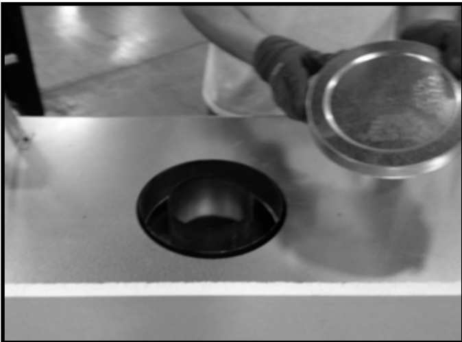
Figure 6.2 Remove the seal cap. (Generic Fireplace Shown)
