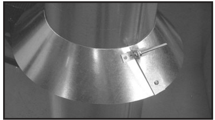
Figure 7.12 Insert Bolt into Brackets
