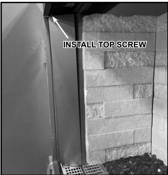
Figure 11.21 Transition Panel installed
