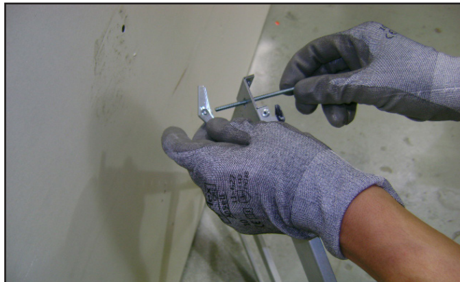
Figure 4.10 Toggle Bolt Installation through Mounting Bracket
