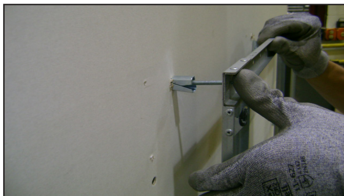
Figure 4.11 Installing Anchors in Hollow Wall
