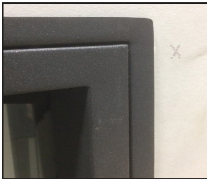
Figure 4.7 Front / Trim Ring Installed to Overlap Wall
