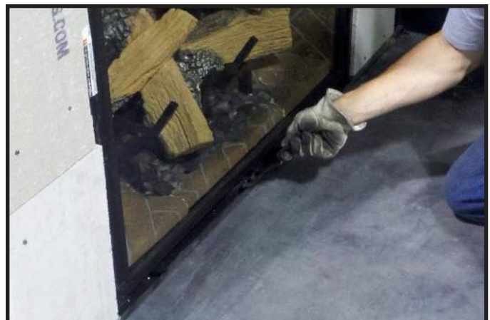
Figure 11.8. Securing Bottom Glass Clips
