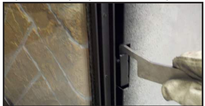
Figure 11.7. Securing Side Glass Clips
