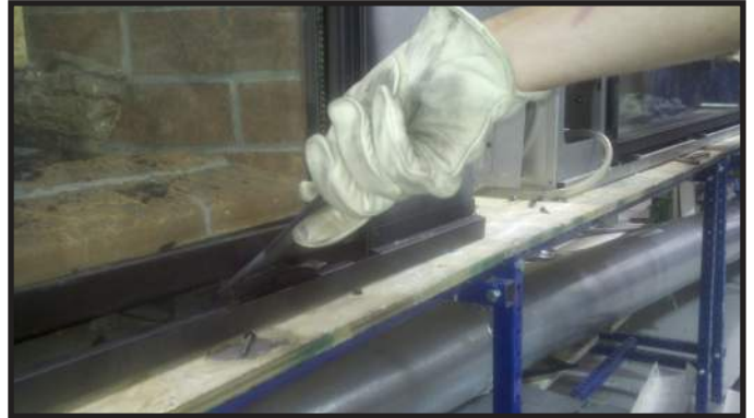
Figure 11.3. Inserting Glass Clip Tool
