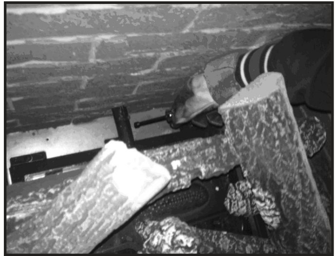
Figure 1. Air Shutter Location
