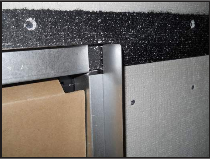
Figure 10.5 Finishing Template Bends
