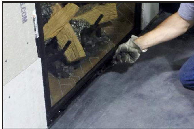
Figure 11.8. Securing Bottom Glass Clips
