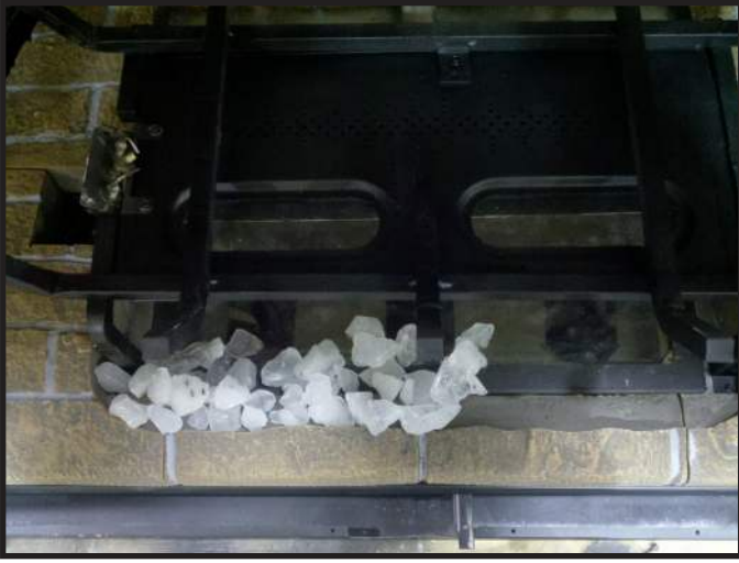
Figure 11.19. Install Teco-Sil
