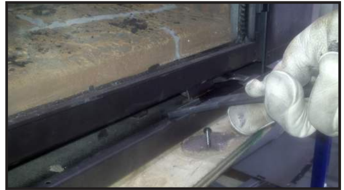
Figure 11.2. Glass Clip Tool Location
