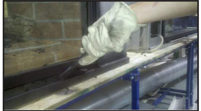
Figure 11.3. Inserting Glass Clip Tool
