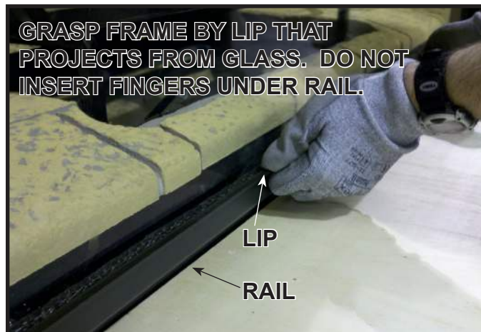
Figure 11.6. Installing Glass
