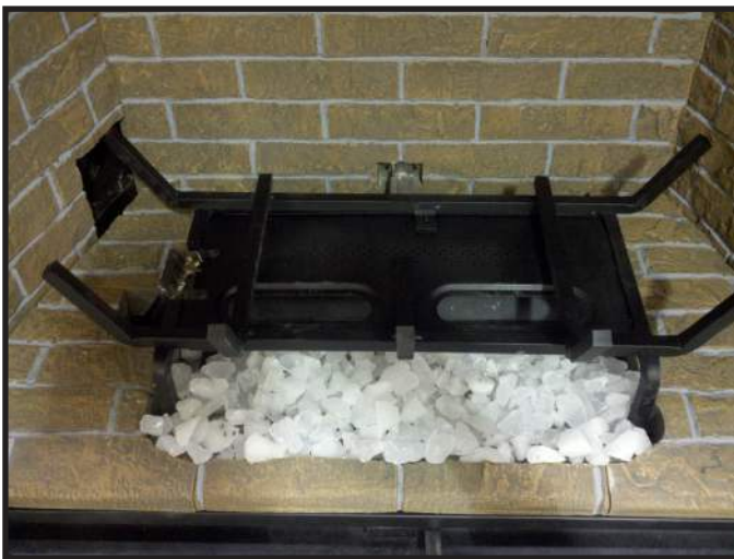
Figure 11.20. Ember Glass Area Covered with Teco-Sil
