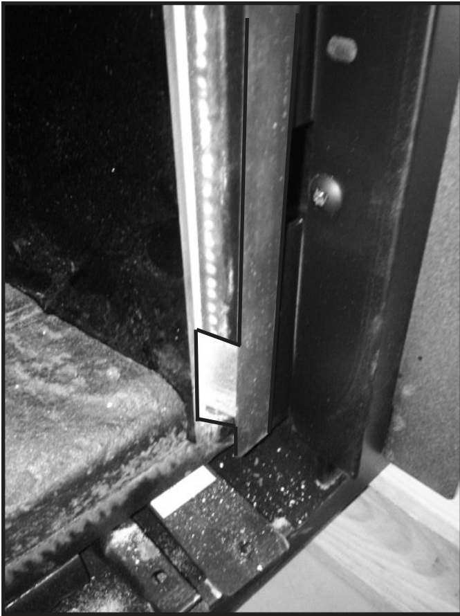
Figure 11.17 Lower Right Finish Trim
