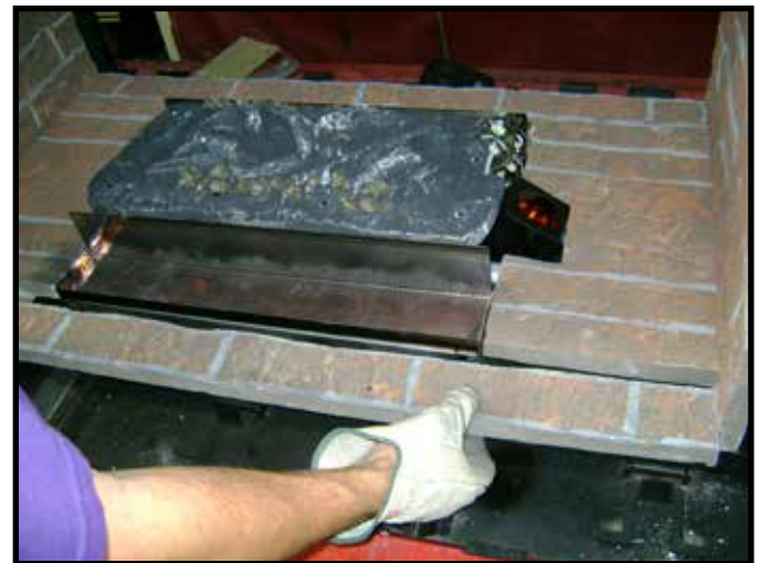
Figure 11.19 Positioning Outer Bottom Refractory.
