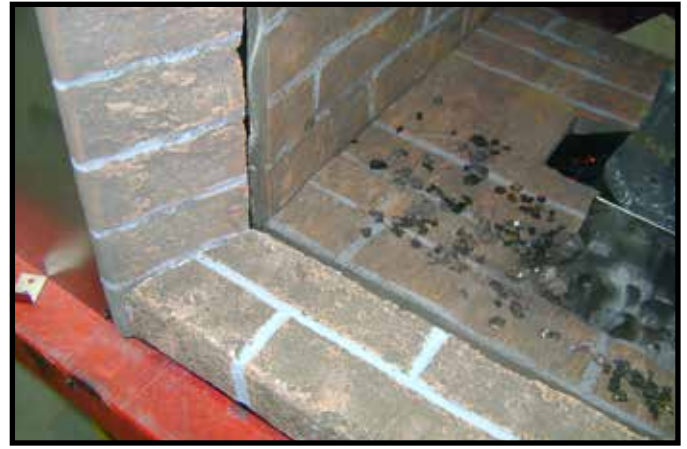
Figure 11.28 Outer Hearth Installation
