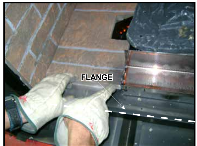
Figure 11.18 Positioning Left and Right Middle Base Refractory
