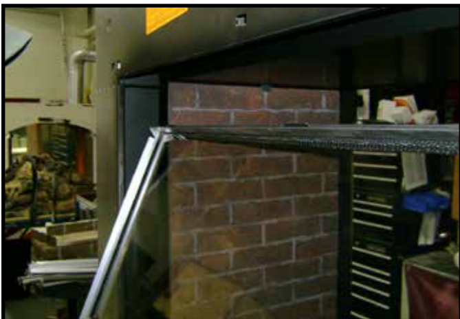
Figure 11.2 Initial Positioning of Frame into Opening.
