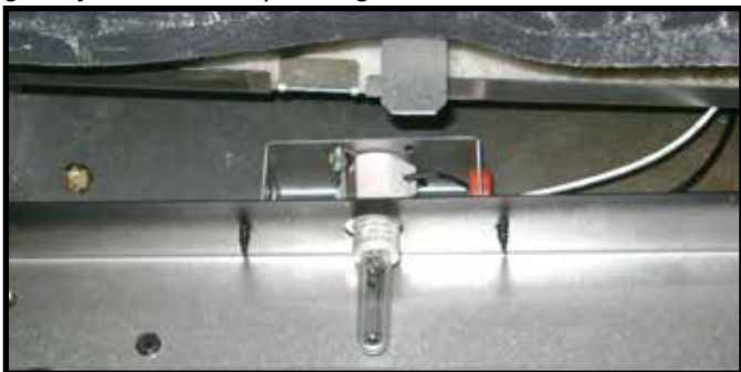
Figure 11.10 Ember Light Bulb Installed
