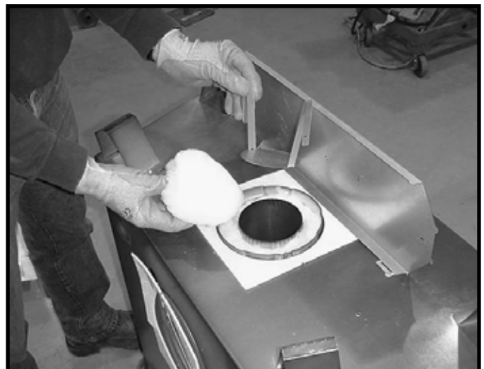
Figure 6.9 Remove the insulation basket and white insulation from the center vent pipe.
