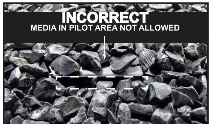
Figure 9.11 INCORRECT Media Placement
