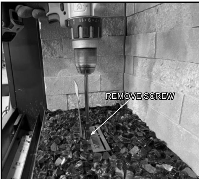
Figure 11.4 Place Media, Remove Media Placement Jig Screw
