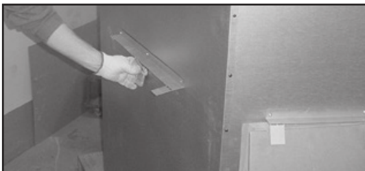
Figure 3.7 Bending Refractory Shipping Tabs Back Down
