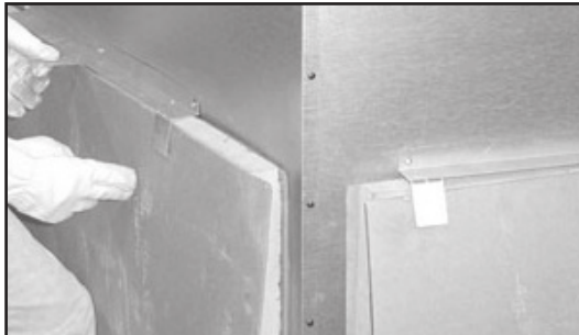
Figure 3.6 Unpack Back Refractory
