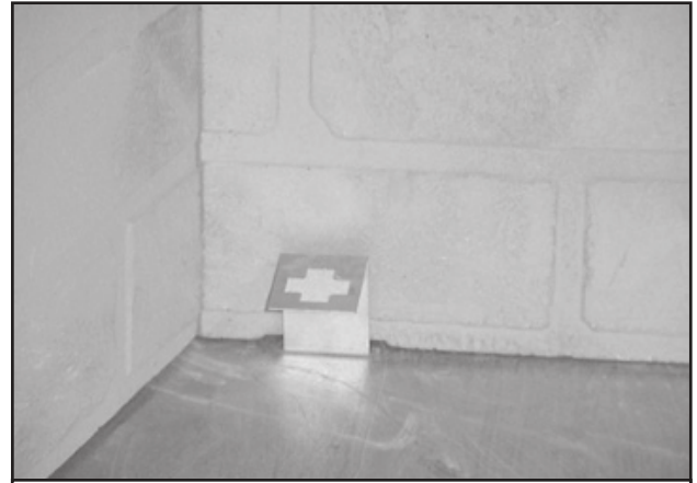
Figure 8.8 Grate Retaining Bracket in Place
