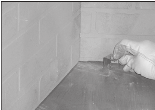
Figure 8.7 Slide Grate Retaining Bracket into Notch
