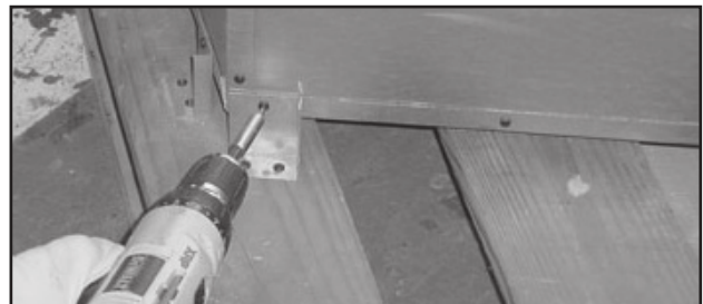
Figure 3.11 Removing Shipping Brackets
