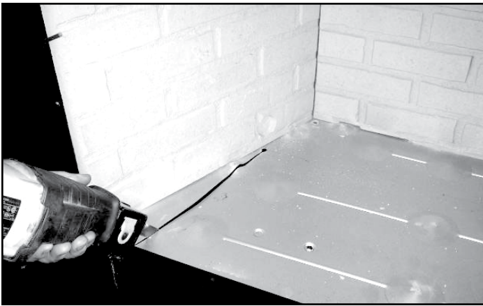
Figure 12.1 - Using a saws-all, cut out the floor.
