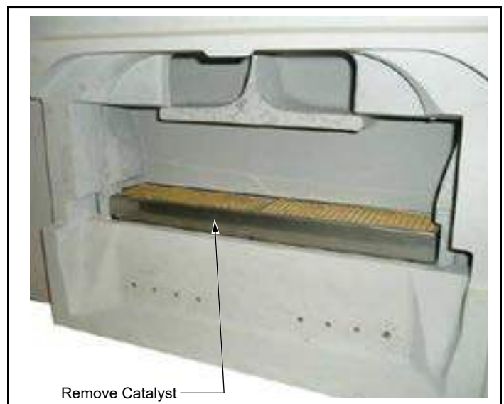
Figure 3.12 - Remove catalyst.
