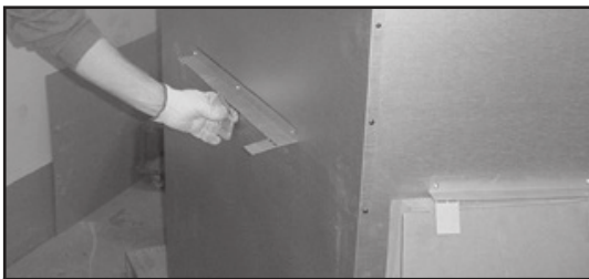
Figure 3.7 Bending Refractory Shipping Tabs Back Down
