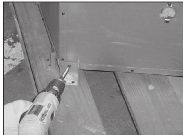
Figure 3.12 Removing Shipping Brackets
