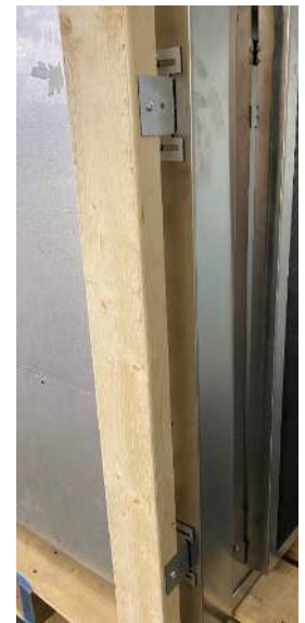
Figure 6.8 Fasten installation brackets to wall framing
