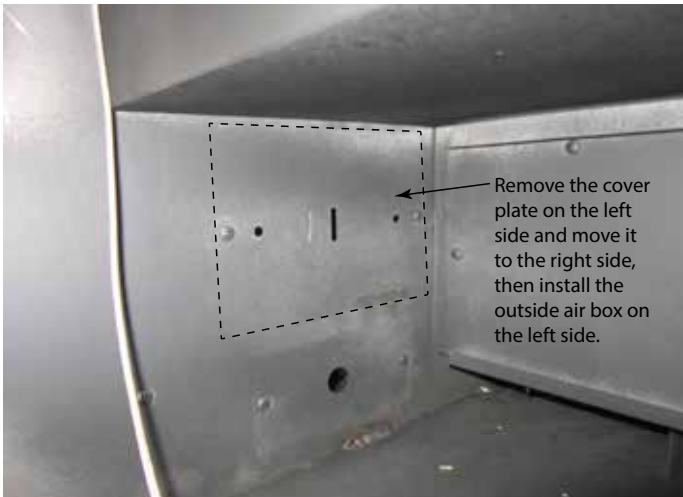
Figure 3.14 Remove Cover Plate (Left Side)
